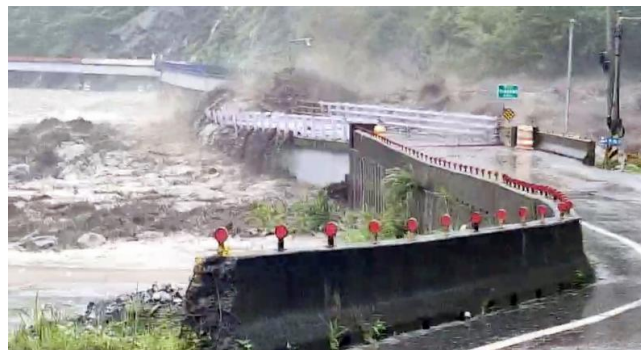
Yusui River bridge, Kaohsiung's Taoyuan District.
